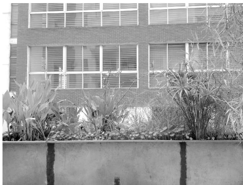
Figure 10.7 (a) Schematic diagram of HSSF systems; and (b) photograph of HSSF systems.
