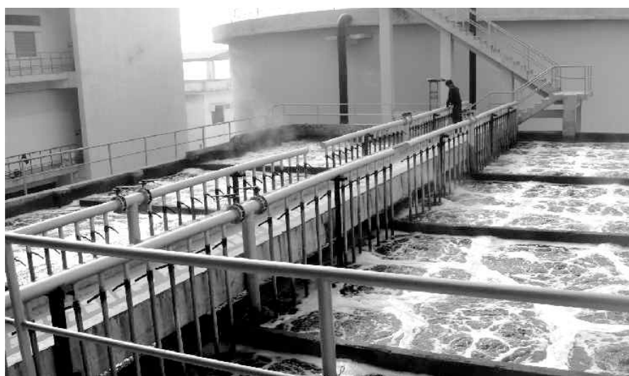
Figure 8.9 Combination of anaerobic digester-aerobic treatments for dyeing effluent treatment in Bangladesh.
